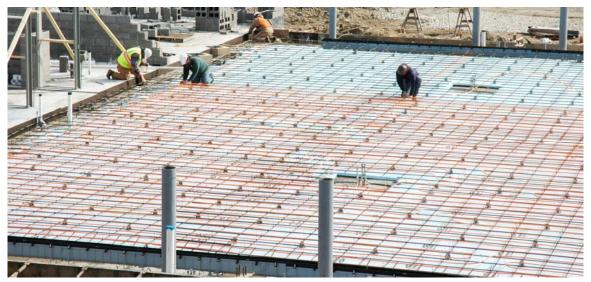
Construction workers install tubing/piping that will help distribute geothermal heating and cooling in Mid-South Community College's \$9 million Renewable Energy Center.
